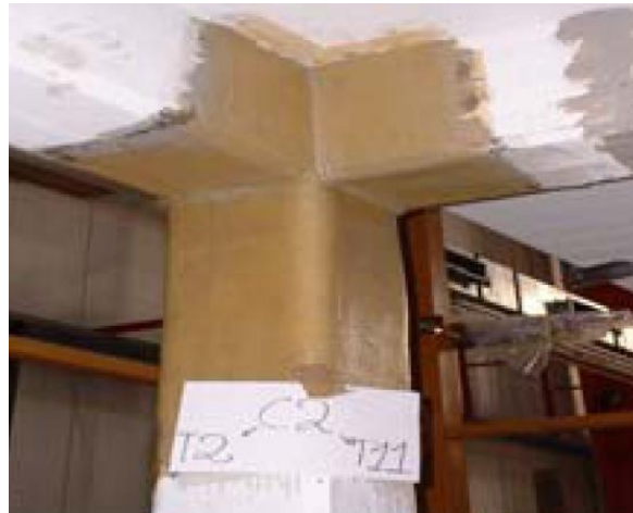
Figure 2. Retrofitting with FRP.
