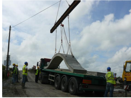
Figure 2b Arch unit during lifting
