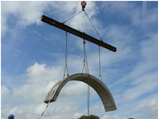
Figure 2c Transfer to bridge location
