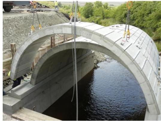
Figure 2d Locating unit on precast sill beams
