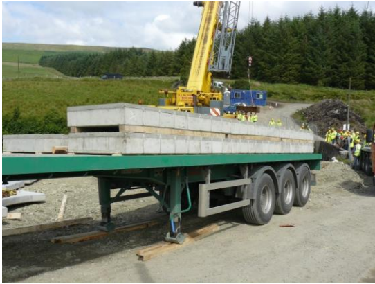
Figure 2a 'Flat-Pack' arch system
