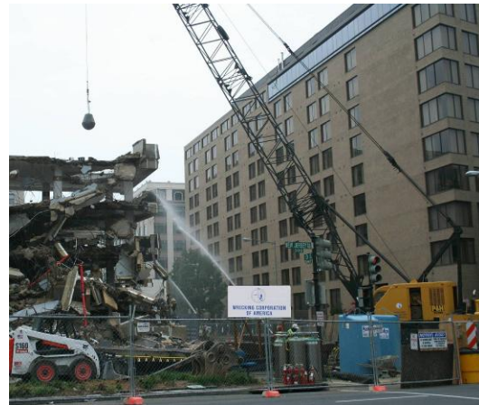
Figure 5. Example of progressive demolition as alternative solution techniques in end of life management ( http://www.wreckingcorp.com ).
